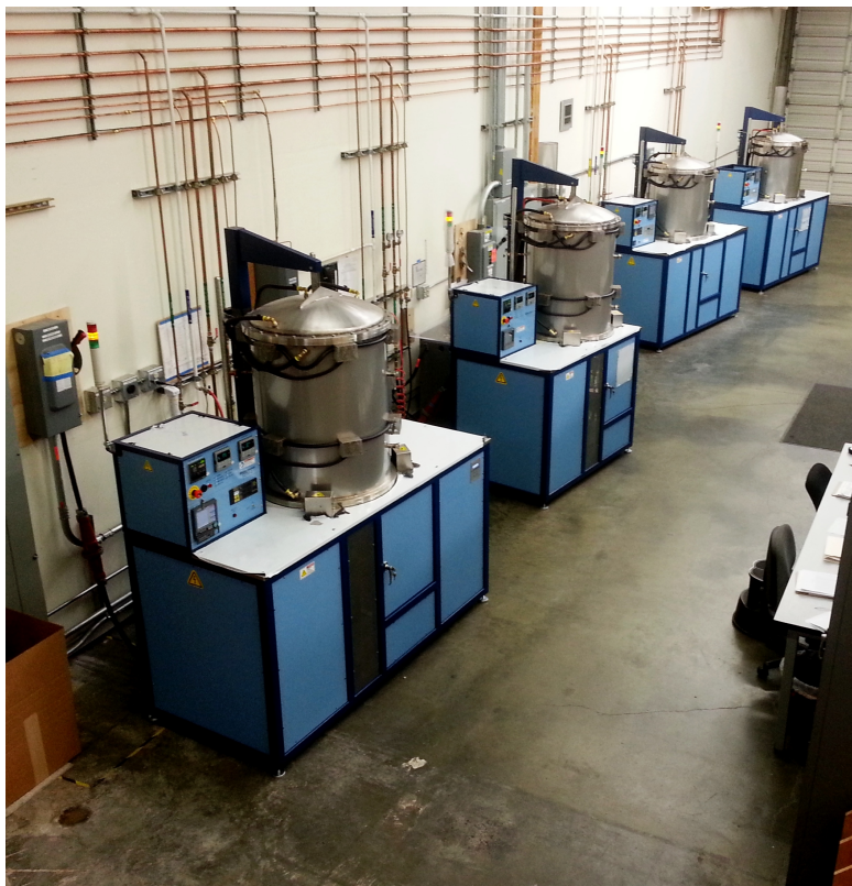
A row of Camco Model 'J' Furnaces at their test facility in San Carlos, California.
